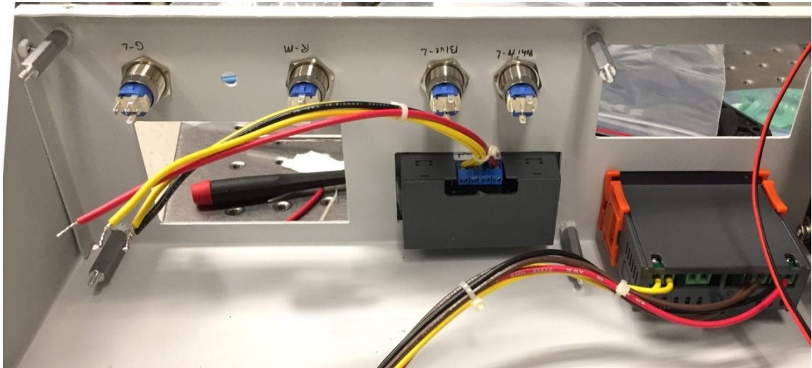
Inverted Top Section, Control Panel Cluster inside View During Assembly
