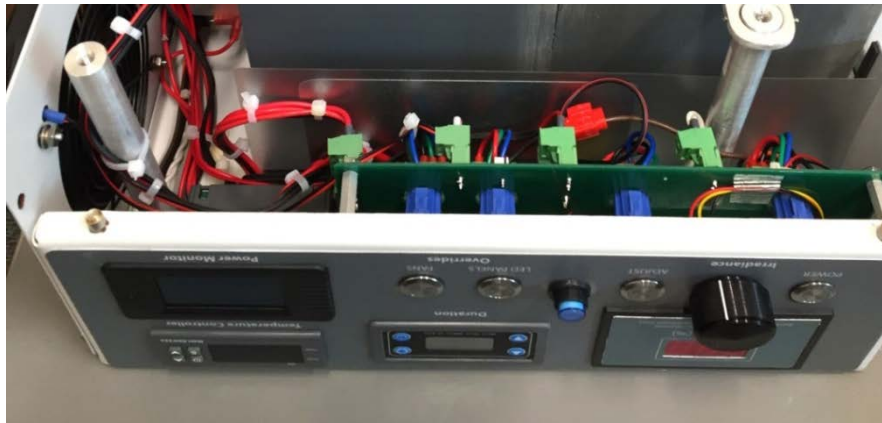
Inverted Top Section Showing PCB Relative to the Control Panel
