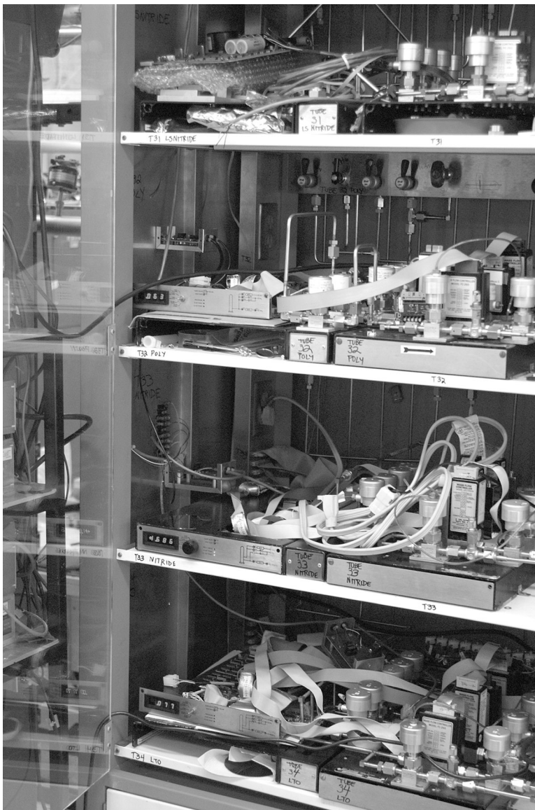
Figure 2.43 Mass-flow controllers for the LPCVD system.
